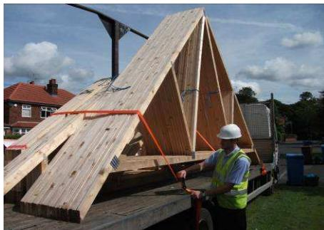
7. The driver will then separate each truss at the heel by placing a wedge between the first and second truss.
