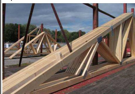
9. The customer team will then take hold of the truss while the driver cuts the blue rope. Once the blue rope has been cut the team will then off load the truss in a safe manner. Proceed with this recommended method for the remaining trusses.
