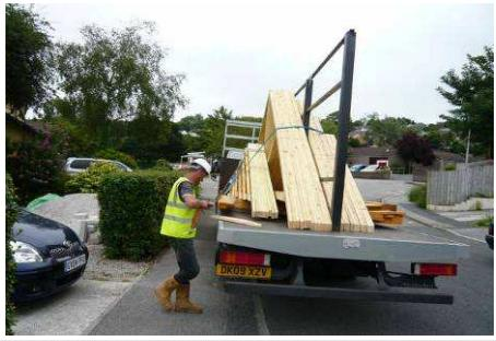
4. The manufacturer will supply truss packs secured to the trailer with blue 3 core rope / banding. You shall familiarise yourself with which rope attaches which pack to the centre bars.
