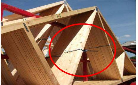
5. The driver will cut the **banding** securing the truss pack to allow separation of the individual trusses. This must be carried out using a closed blade pruning staff.
