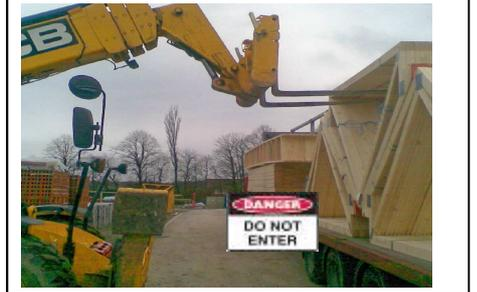
7. The driver will cut the individual rope / banding attaching the pack to the bars. This must be carried out from a safe position using a telescopic cutting staff.
